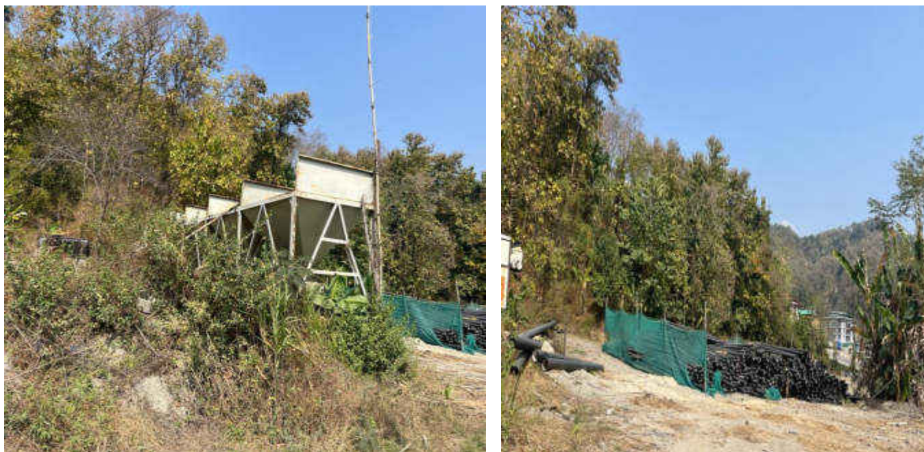
Figure 27: Photograph showing the status of bitumen/crusher plant during site visit
